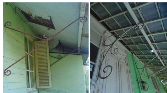
Figure 12. Various types of the schoors. Type 1 in the Residential Houses of Military District Commander (left), and type 2 in the Residence of Military District Command Staff Chief (right). Source: Hasrianti, 2017.
