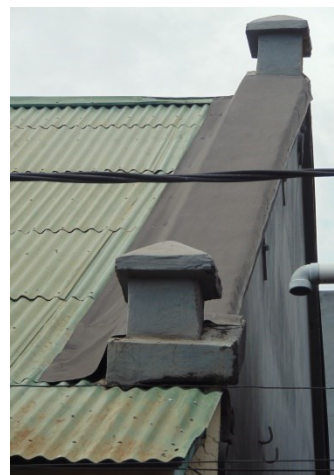
Figure 10. The geveltoppen in Chinese Shophouses. Source: Hasrianti, 2017.
