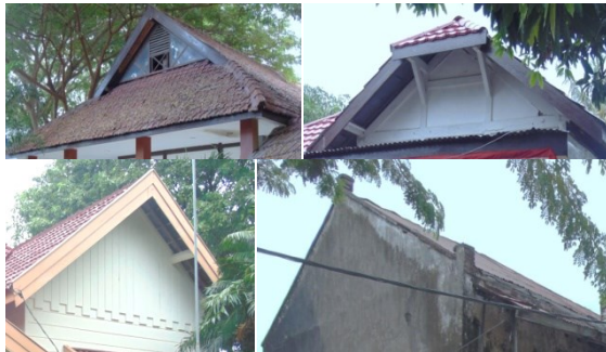
Figure 4. The Dutch gable on Guest House (top-left), the jerkinhead gable on the Residence of Police Resort Chief (top-right), the open gable in Colonial Building 1 (bottom-left) and Chinese shophouses (bottom-right). Source: Hasrianti, 2017.
