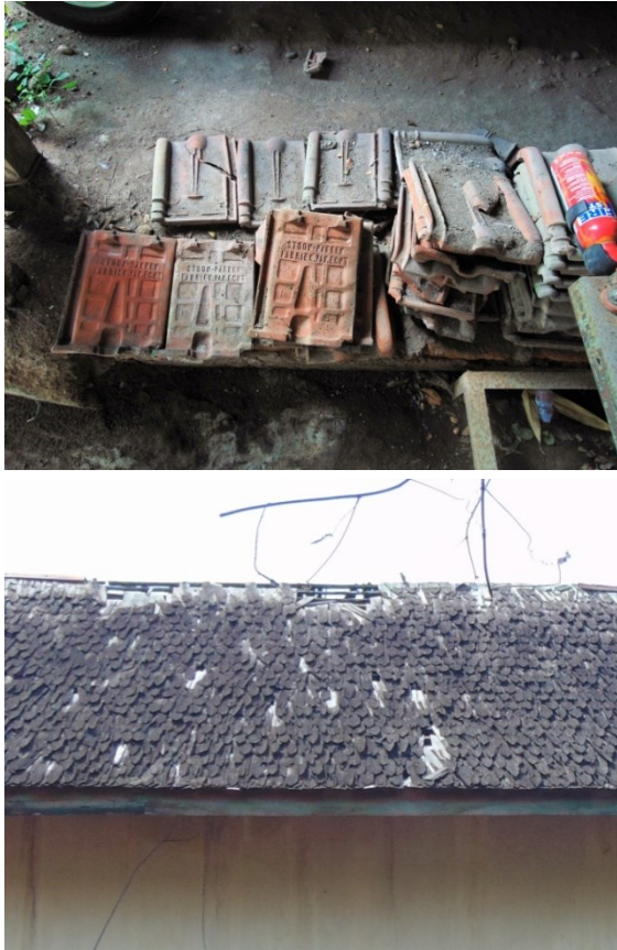
Figure 2. The various of roof materials, above: clay roof tiles, and bottom: shingle. Source: Hasrianti, 2017.
