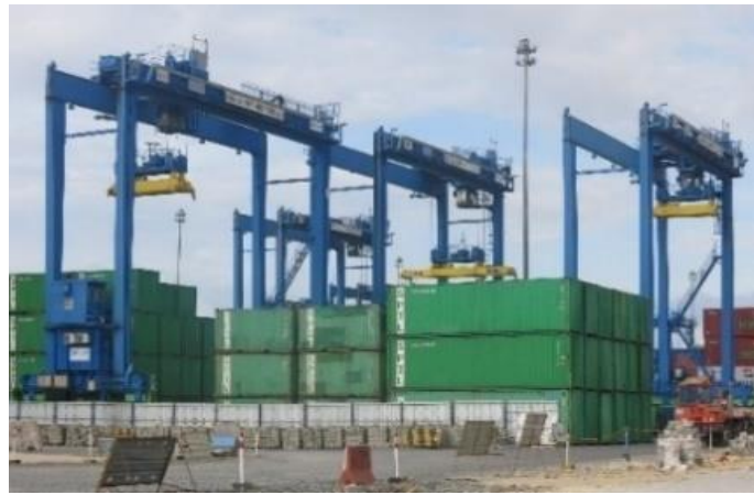
Figure 7. Eksisting Rubber Tyred Gantry (RTG) dan Container Yard Terminal II of the New Makassar Container Port
