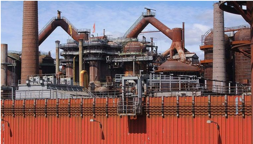
Fig. 1. Industrial Corrosion Area
